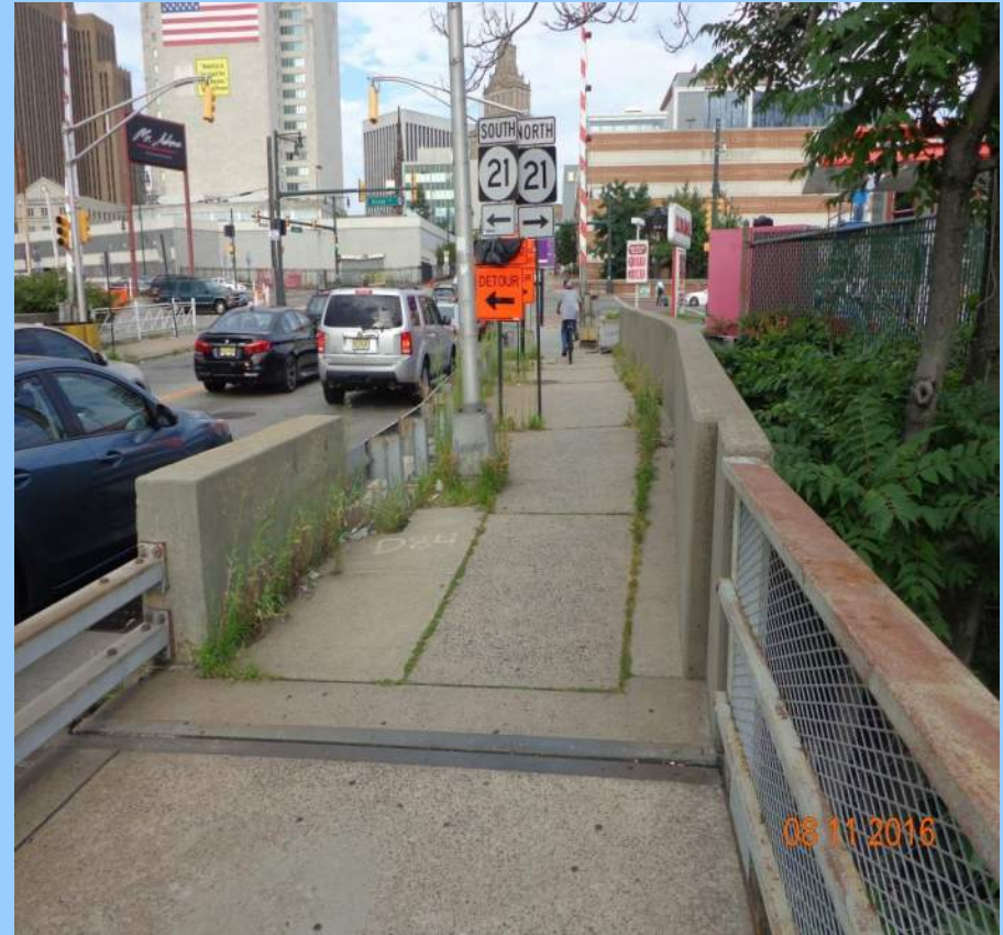
West Approach to Bridge looking towards McCarter Highway
