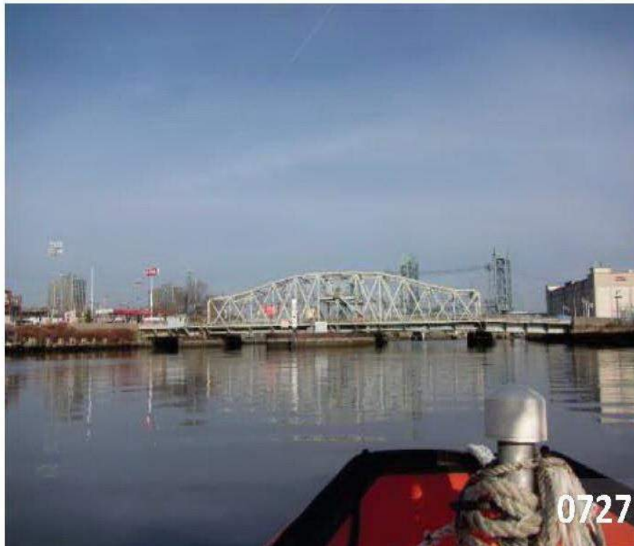
South Elevation Looking North (Upstream)
