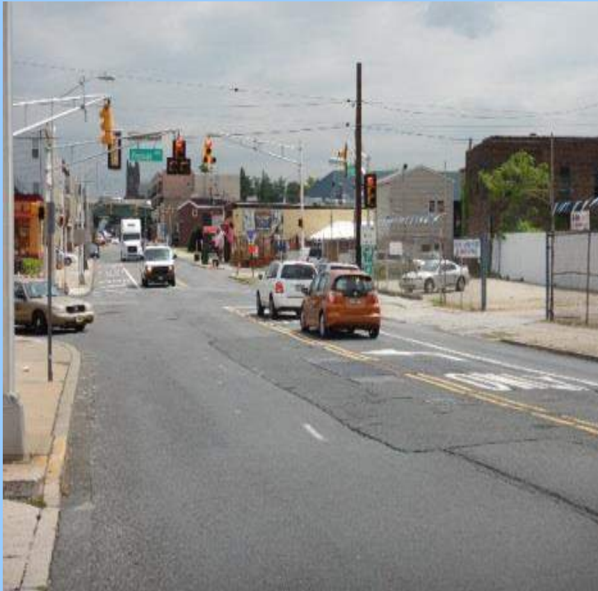
East Approach Roadway looking towards Passaic Avenue
