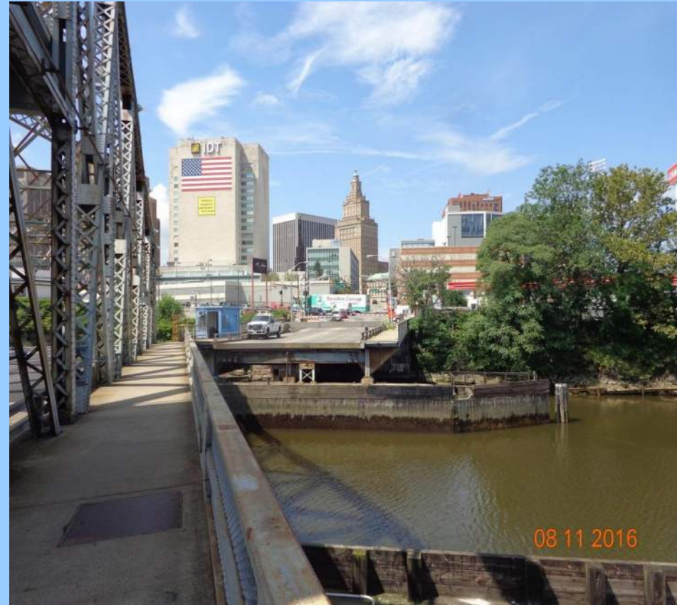
Bridge Opening Looking West at McCarter Highway & City of Newark
