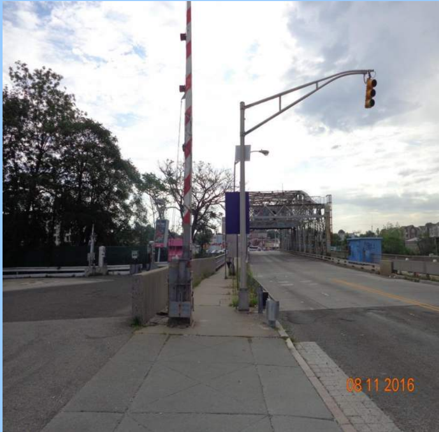
West approach to bridge looking east towards Town of Harrison
