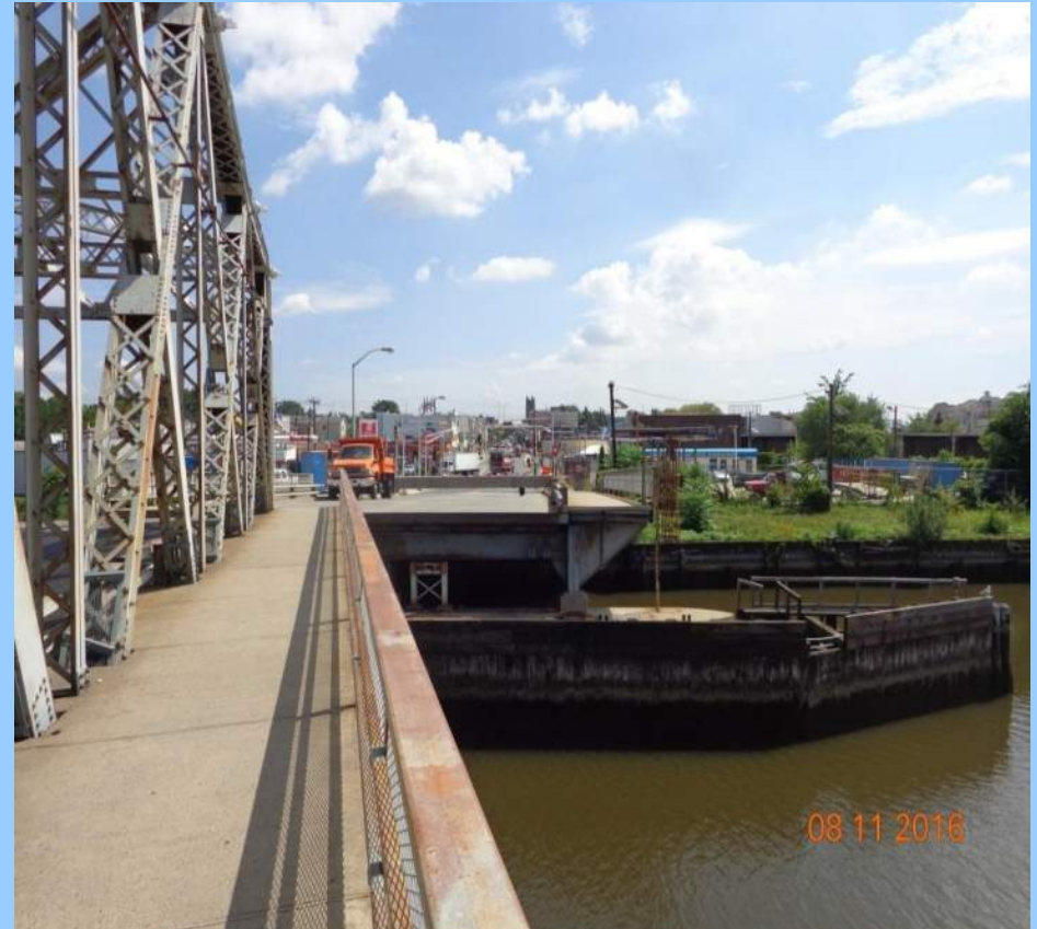
Bridge Opening Looking East at Town of Harrison
